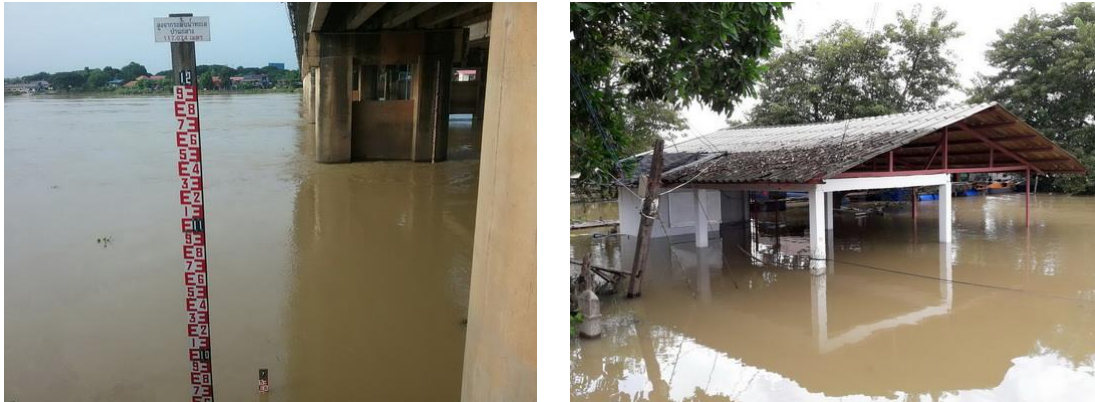
Figure 2 The area after rain and flooding in Ubon Ratchathani Province
